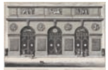
View of the Exterior of the Grotto of Versailles
