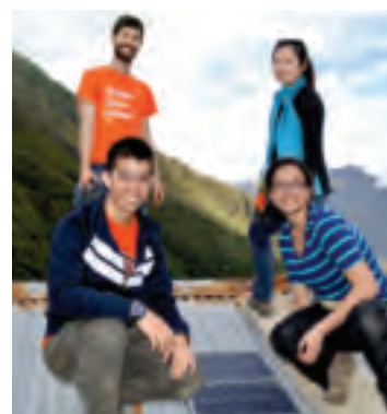
Mark Benjamin '14, Annie Tao '16, Douglas Bastidas '17, and Jackie Rambarran '16 install solar panels in a remote village in Peru as part of the Pace Center's 2014 International Service Trip.
